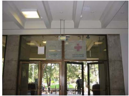
Langsdorf Hall (inside view)
