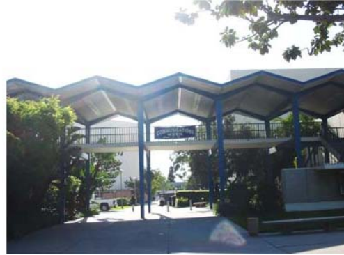
PA – McCarthy Hall – Building Bridge
