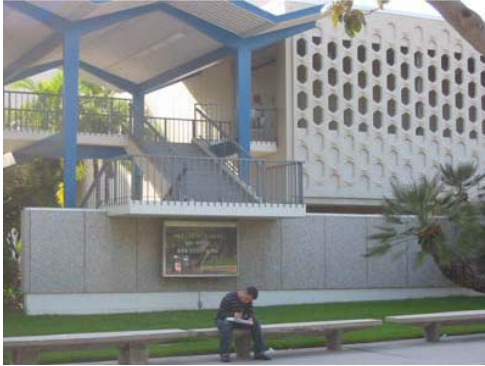
PA – McCarthy Hall – Building Bridge
