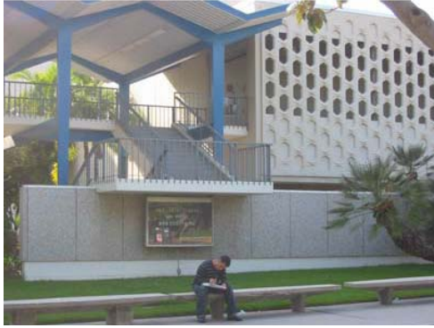
PA – McCarthy Hall – Building Bridge
