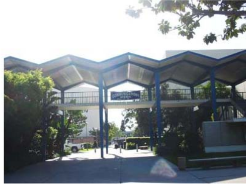
PA – McCarthy Hall – Building Bridge
