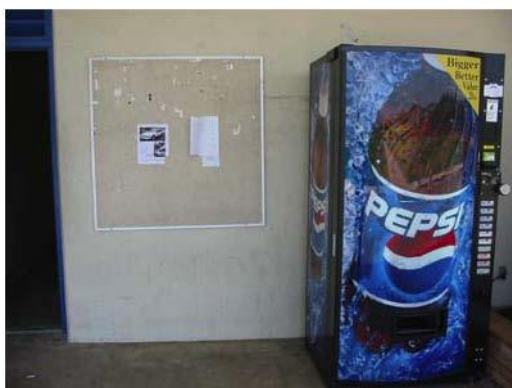
North side of the Kinesiology & Health Science (KHS) building (formerly Physical Education (P) building)
