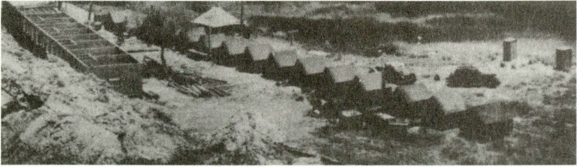
Figure 15. Zzyzx in the 1940s when tents were used and the building called "Sunrise" was under construction.
